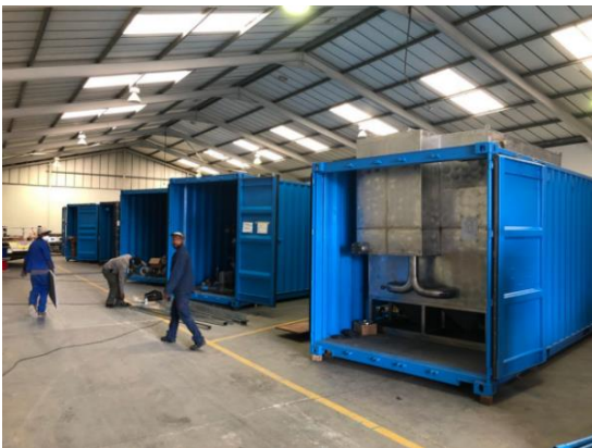
Figure 40: Stellenbosch Containerised WTW being manufactured
